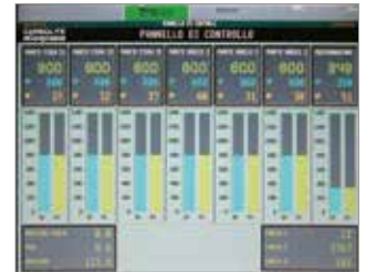
Display showing control zone temperature and setpoint, % power, lance thermocouples, height indicator and wall pressure.
